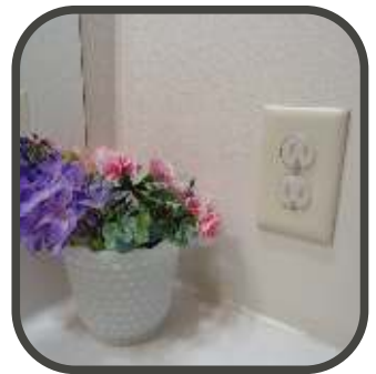
CHILD SAFETY PLUGS ON OUTSIDE- FACING WALLS
