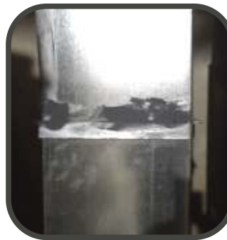
SEALING HVAC DUCTWORK
