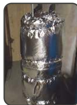
WATER HEATER WRAPPING
