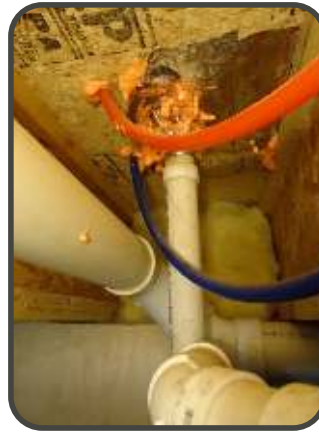
SEALING EXTERIOR PENETRATIONS WITH GAP 'N CRACK
