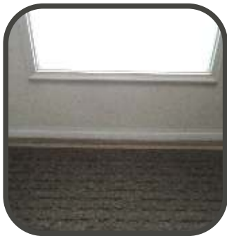
INSTALLED WHITE DOOR- SWEEP ON THE BOTTOM OF THE DOOR
