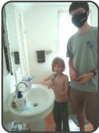
INSTALLING A NEW FAUCET AERATOR
