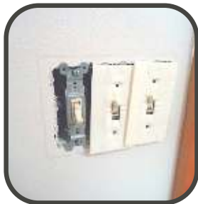
INSULATING PADS ON OUTSIDE-FACING WALLS
